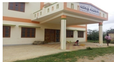
Yatrinivas at Gadidam temple in Chickballapur district remaining unused
